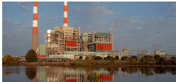
LaCygne Generating Station
