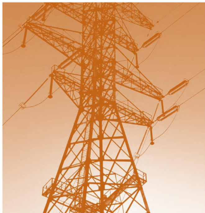
KCP&L and GMO's electric utility system has approximately 3,600 circuit miles of transmission lines
