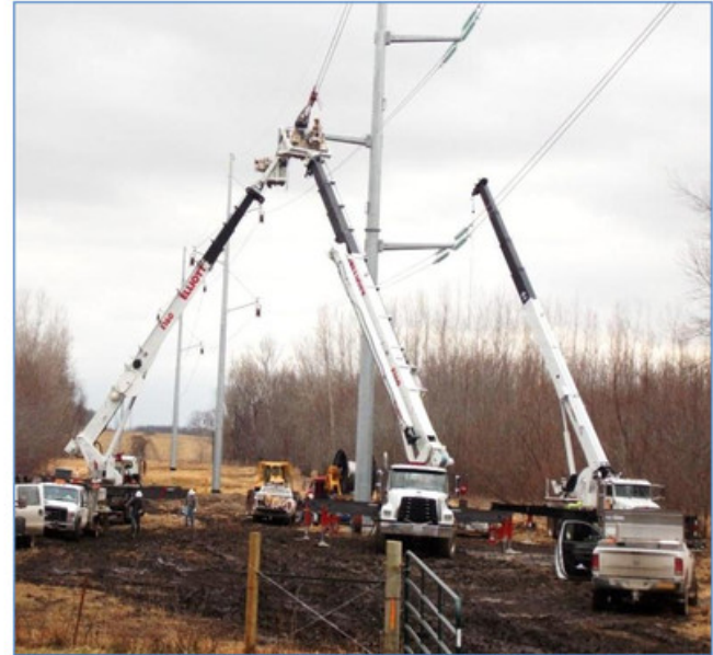
Iatan-Nashua Project under development
