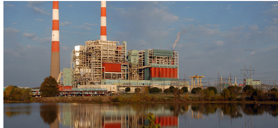
LaCygne Generating Station
